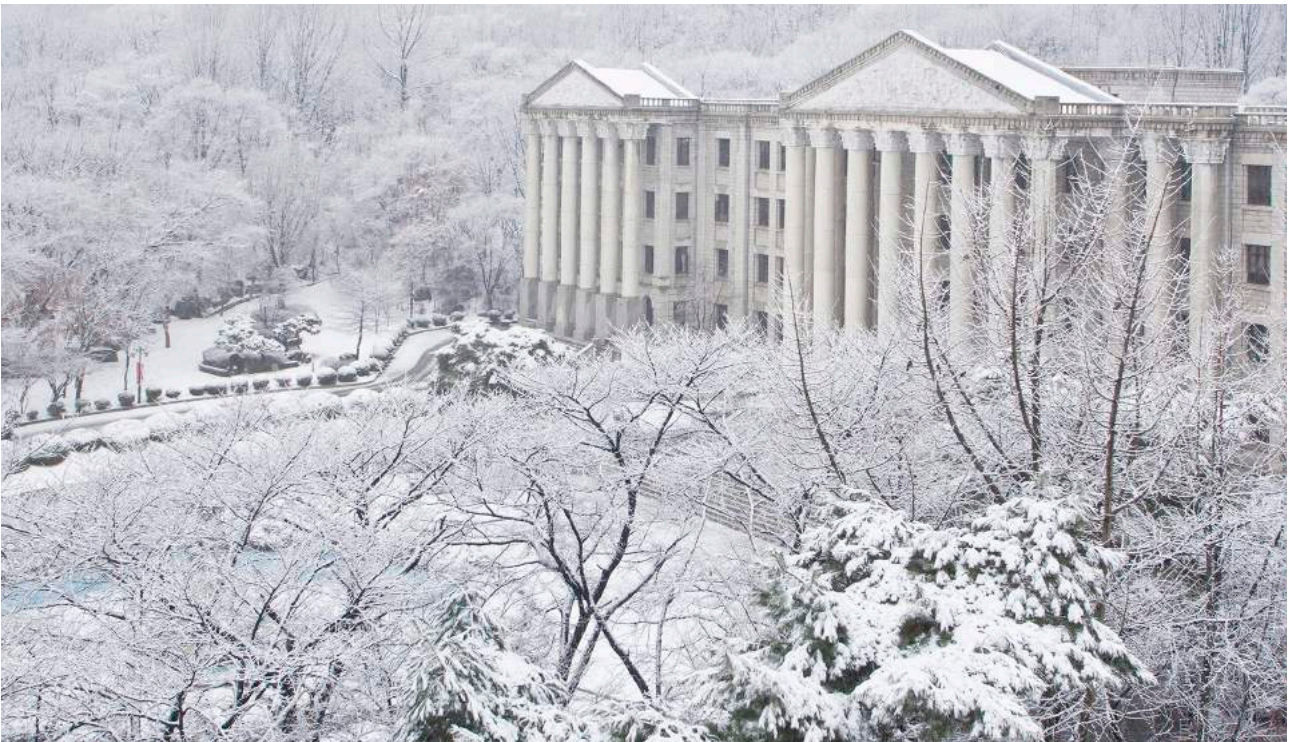
| Winter University Administration Building
